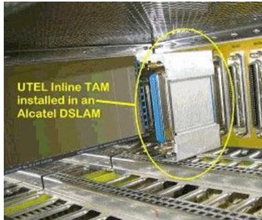
This is the cheapest option for in-line TAM, no additional cables, no extra cabinets, they simply fit into the existing DSLAM rack. Partial installations are also possible, adding additional modules as the customer base expands.
